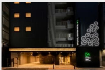
karaksa hotel TOKYO STATION
